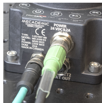
(c) Connectors properly attached
